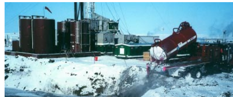
Sump in the Mackenzie Delta Photo Source: Newpark Environmental Services
